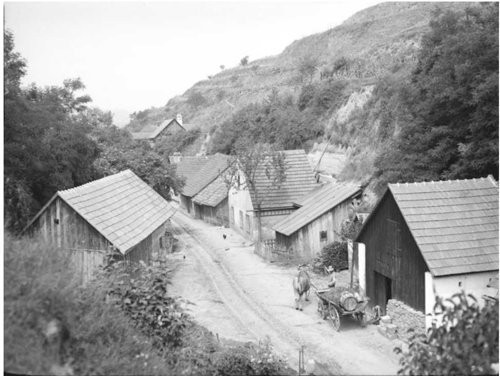
Fig. 11.8 Cellar lane in Wagram ob der Traisen (close to Traismauer) around 1925. Note the ox drawn cart, the incised tracks on the soil surface of the sunken road, the steep loess slopes, and the press houses built right next to the walls covering the entrance to the cellar tubes. Source ONB/Vienna, Picture Archives 57.515-B
