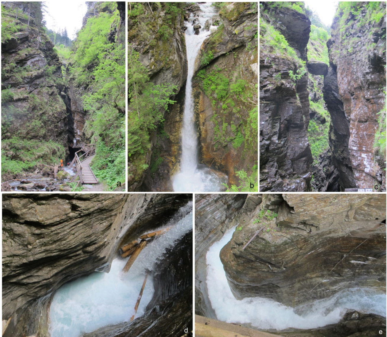
Fig. 26.5 Above from left to right: a a view of the emerging Ragga channel shows that the slot profile stands up clearly from a steep V-shaped gorge; b the head of the gorge, a 17 m high waterfall-step into resistant pegmatites; c a trapped boulder between rock ledges about
