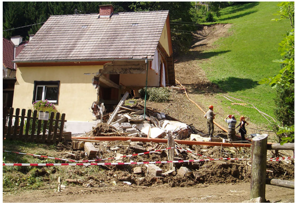
Fig. 6.5 Landslide in Gasen/Haslau, Central Alps, c. 35 km northeast of Graz, in August 2005. Picture credits Arben Koçiu, Austrian Geological Survey, with permission
