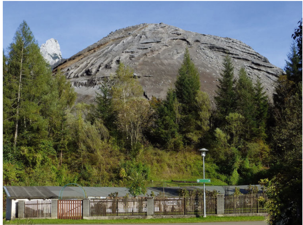
Fig. 30.9 Slagheap of M \ddot{u} nichthal. It was emplaced between 1901 and 1946, consists of 1.8 Mio m 3 of slag, with a basal diameter of 300 m and a height of 65 m (Bundesministerium f \ddot{u} r Nachhaltigkeit und Tourismus 2012). Publicly available Google Photo
