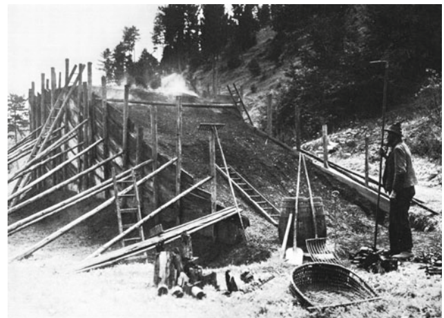
Fig. 30.3 Rectangular charcoal kiln set up and operated by the local peasant population as supplementary income opportunity. This charring method, as shown in the image taken around 1940, was practised basically unaltered for centuries (Hafner 1979)
