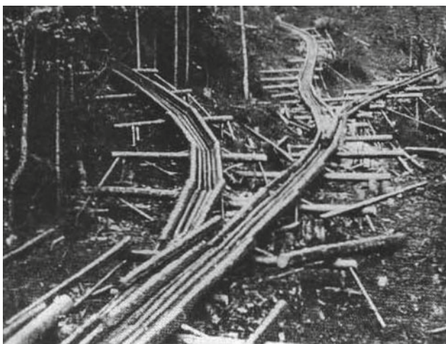
Fig. 30.4 Wooden log slide around 1923 in a tributary canyon of the Enns Valley debouching c. 8 km west of the Erzbach. Log slides were constructed since the late thirteenth century to transport massive amounts of logs downslope to the river systems (Hafner 1979)
