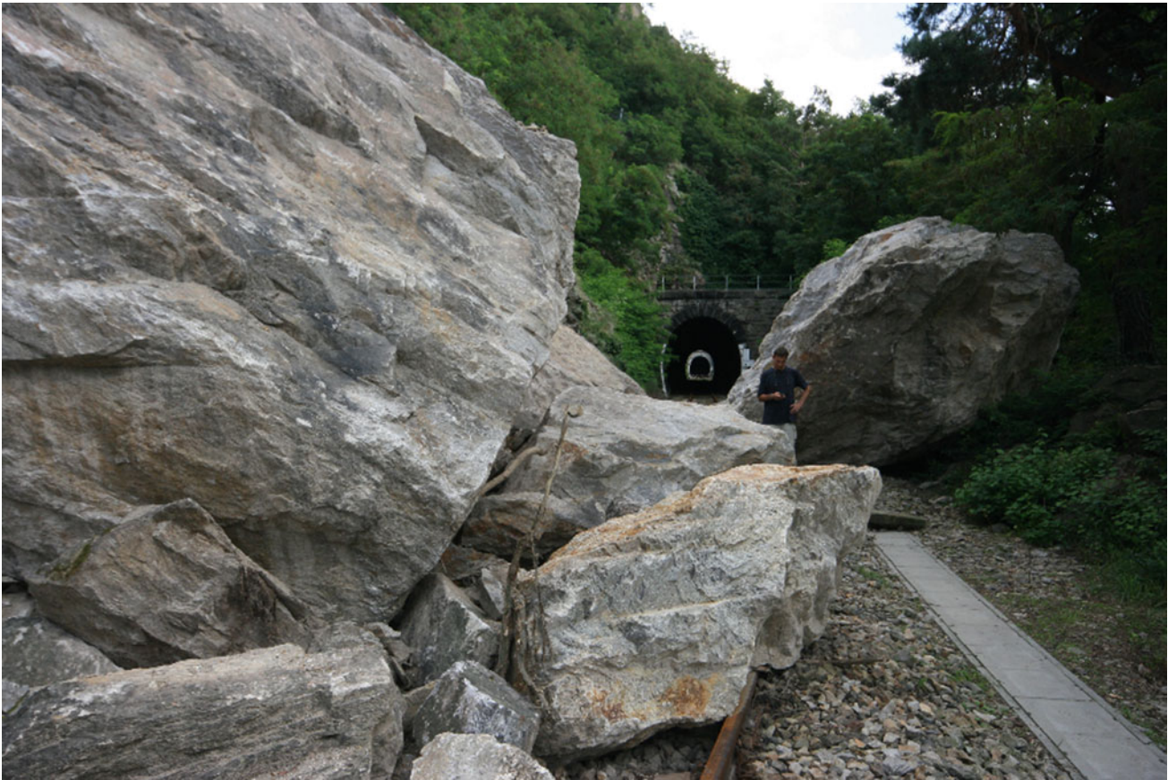
Fig. 10.15 Rock mass fall from the Biratalwand at Dürnstein in July 2009, destroying the track of the Wachau railway. Photo: R. Roetzel
