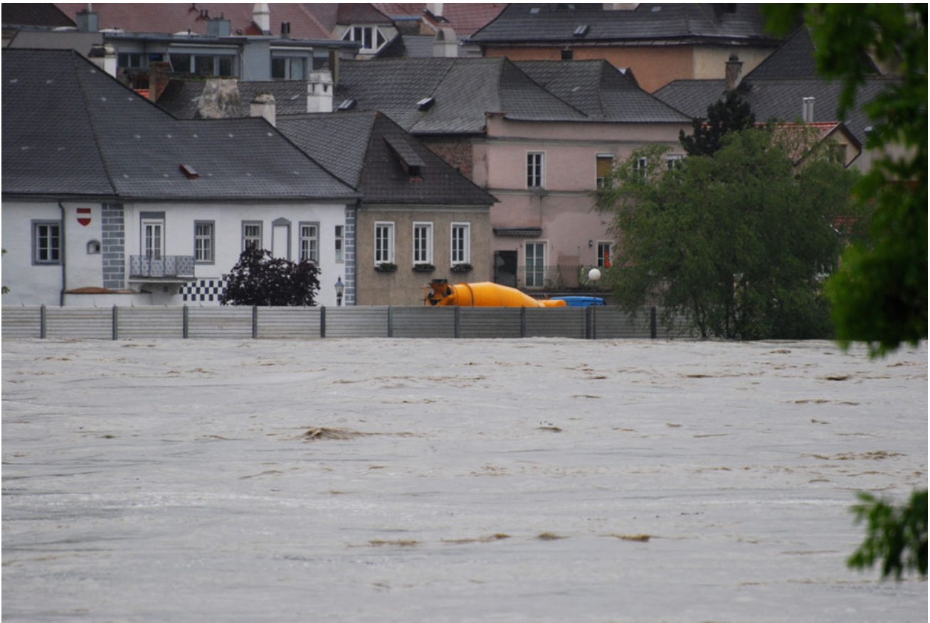
Fig. 10.13 Mobile flood protection structures along the river banks of the Danube in Krems-Stein during the HQ 100 event on June 3rd 2013 in Krems-Stein. Photo: R. Schmid
