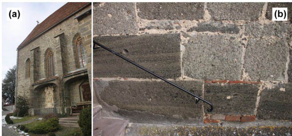
Fig. 33.6 An example of the use of volcanic rocks in the study region for construction purposes. The church of the settlement of Riegersburg (a) is made of basaltic tuff (b), which was quarried from the nearby
