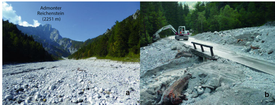
Fig. 18.10 Sediment transport in the Zwischenmüer area. a View of the gravel bed in the Langgriesgraben in SW direction. b Example of a debris flow that was dammed by an undersized bridge opening and
